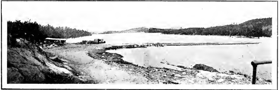
WANAPITEI LAKE STORAGE—SUDBURY DISTRICT Looking upstream from end of main dam; old dam in centre of view
